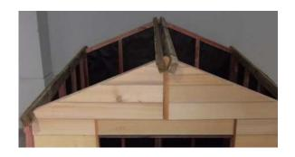
Step 14: Using 1 x 75mm tek screw, screw bottom purlin to top plate centrally in shed.
