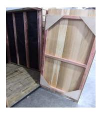
Step 21: Using 3 x 75mm tek screws, screw door stud to panel ensuring height is correct.
