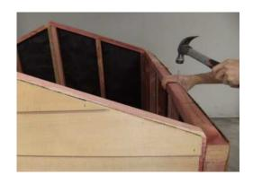
Step 9: Using 30mm clouts nail top cedar boards to stiffeners (2-3 per board). Predrill holes to stop boards from splitting.
